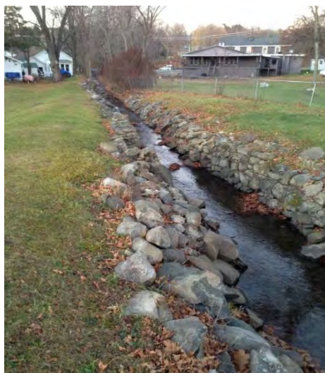
Channel draining Sub-basin 1
