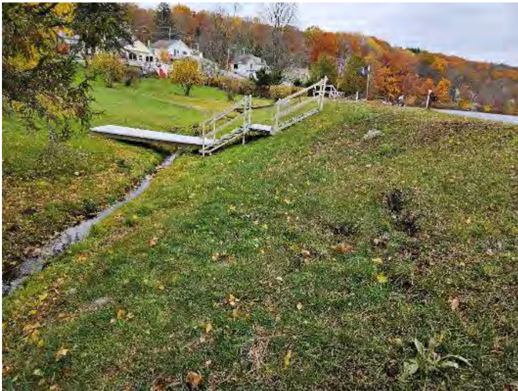
Photo 10: Stormwater ditch at toe of dike. Note recreational features on dike.
