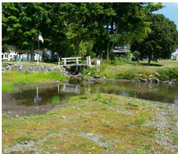
Channel outlet into Glass Lake through the Glass Lake Dike
