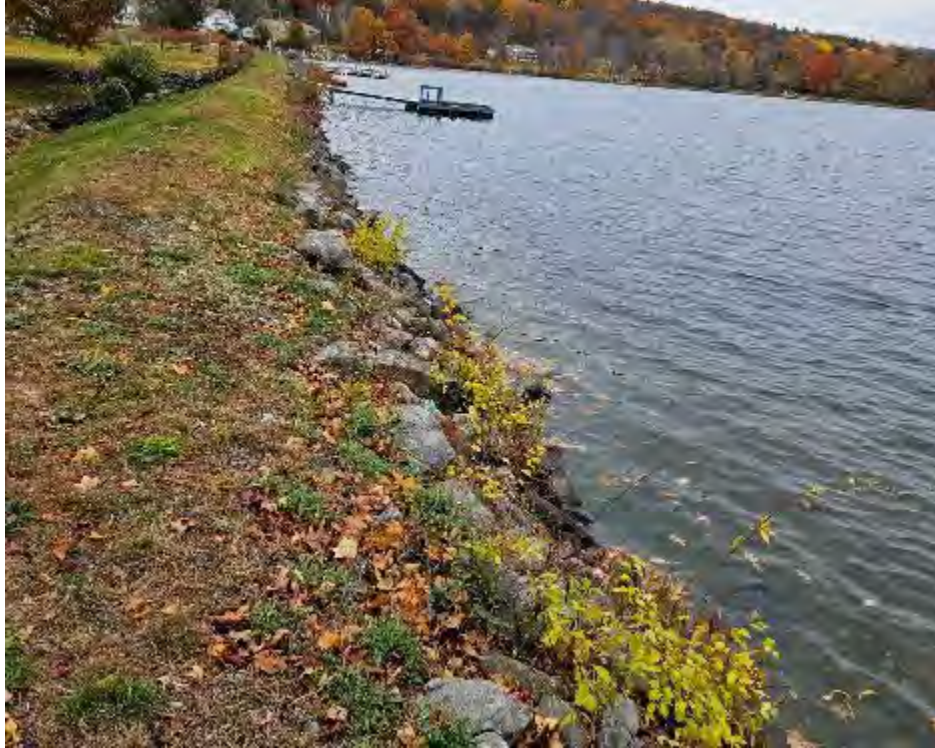
Photo 9: Upstream slope of dike from west end looking east.
