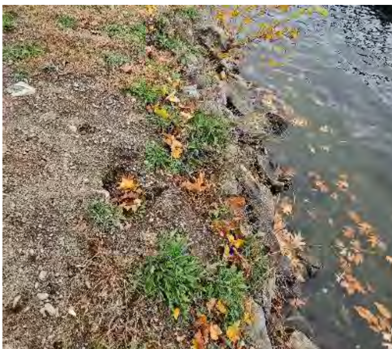
Photo 8: Animal burrow on crest of dike.
