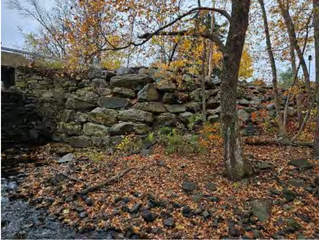
Photo 1: Rock wall on downstream side of right embankment.
