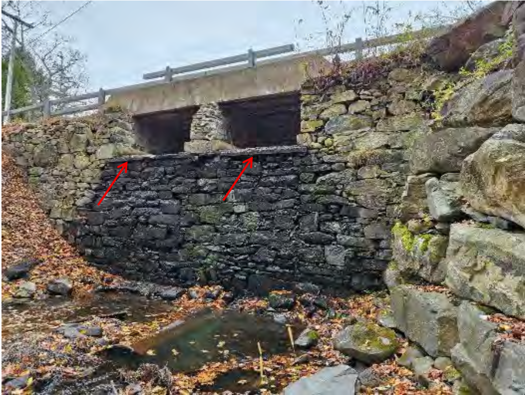
Photo 5: Downstream face of dam. Note wooden planks.
