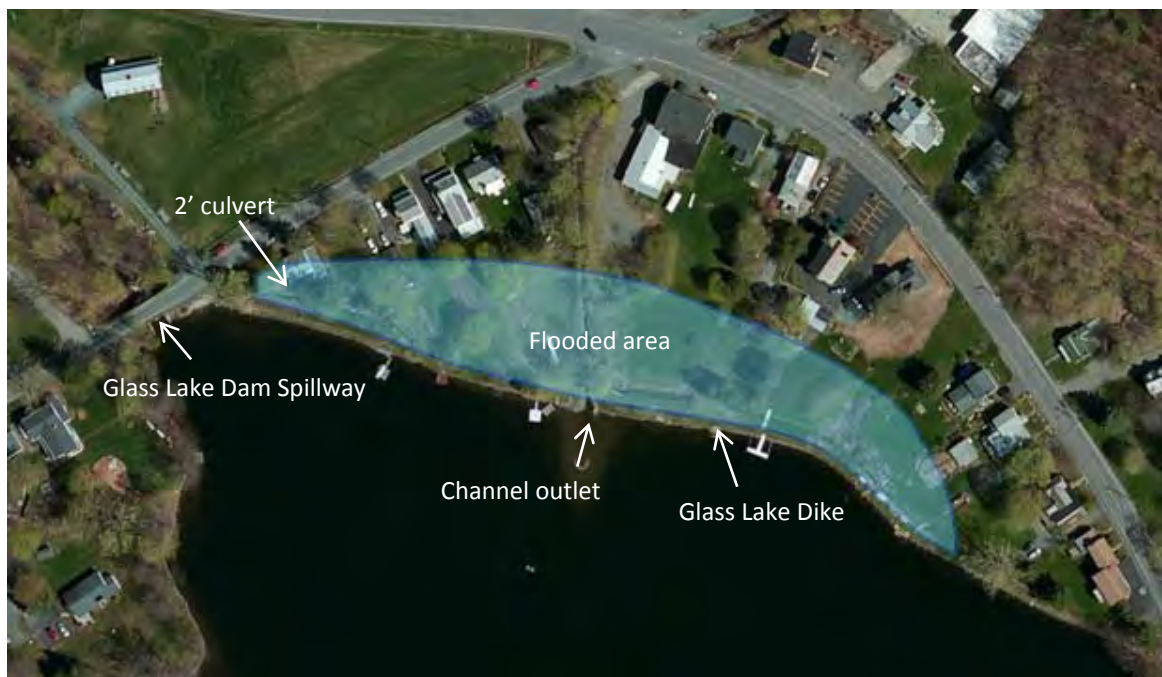
FIGURE 6-2: LOW-LYING AREA DOWNSTREAM OF GLASS LAKE DAM WITH WATER EL. AT 832.3
