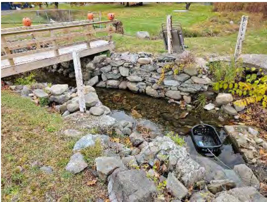
Photo 12: Tributary through dike. Note footbridge.
